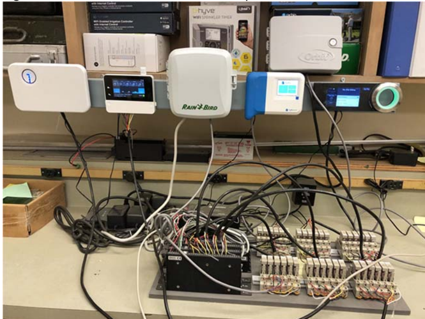
Figure 1. Controller installation and Setup in the Lab
