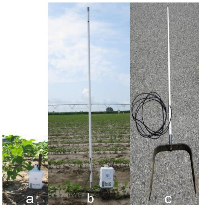
Figure 2. (a) Em50G logger installed in cotton field; (b) Em50R logger with the antenna mount in soybean field; (c) Antenna mount.
