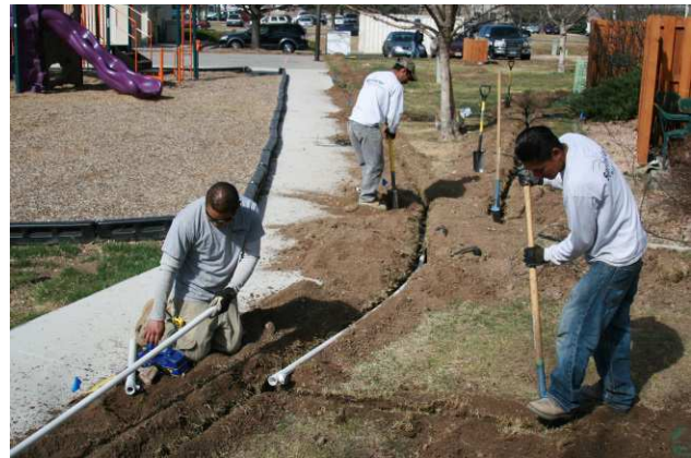
Installing a sprinkler system
