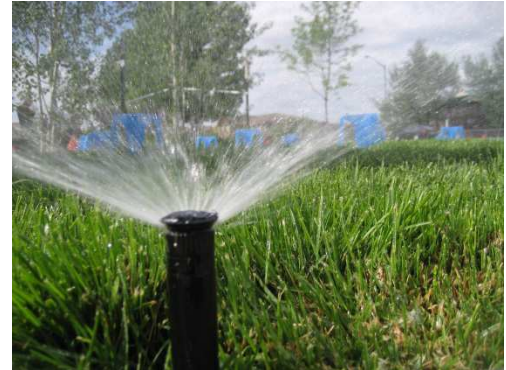
Sprinkler head with catch cans
