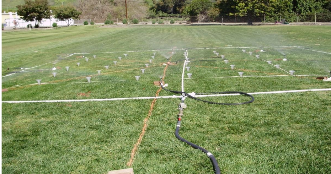
Figure 1 Irrigation system for testing nozzles with catch can grid.
