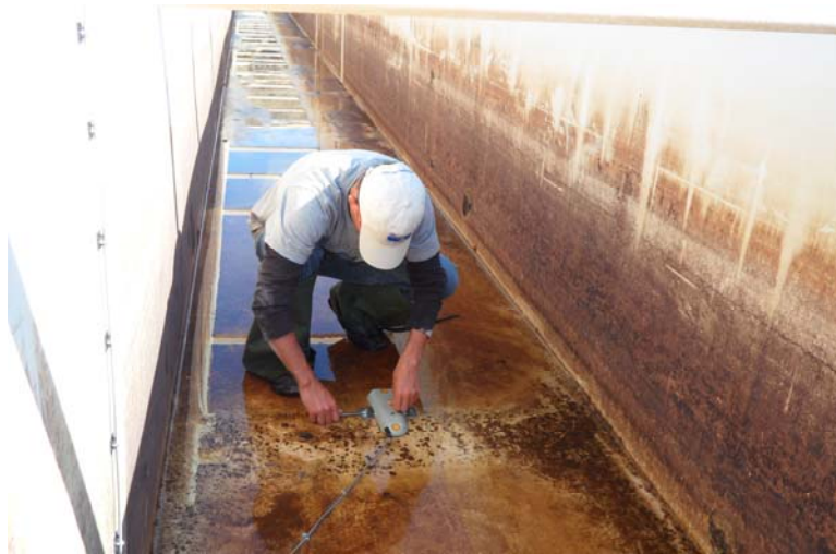
Figure 2. SonTek IQ installation at ITRC flume
