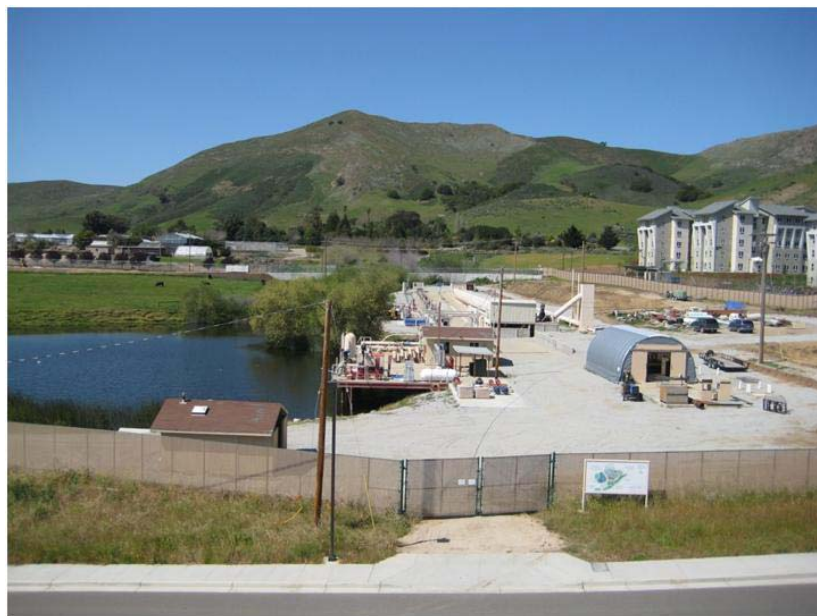
Figure 1. California Polytechnic State University - Irrigation and Training and Research Center
