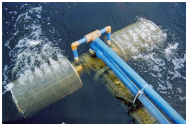
Figure 1: Pump intake screen
