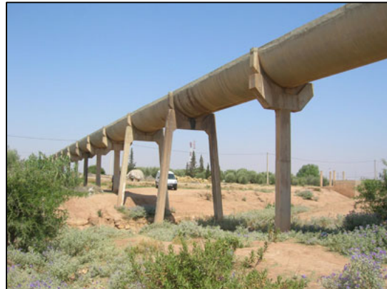
Figure 4. Raised irrigation canal at PIT. Source: ORMVAT
