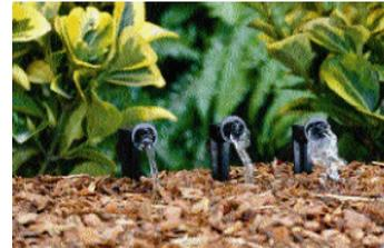
adventurous and will slowly become the norm. Coated in root inhibitor the old saying that roots followed the water into the emitter and stopped the flow is now old school. Surface installed dripline spaced in a triangular layout with distance dictated by soil type is used to flood irrigate mass planted areas. Tree root watering systems utilizing micro-bubblers are available to deep root water
