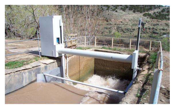
To counteract this lift force, the bottom beam of the gate was securely anchored to the concrete stem-wall and the upstream side plates were bolted to the concrete side walls. The greater hydrostat force across the gate-leaf required high inrush current to the motor to start the gate moving. Because of increased the inrush current through the motor, the DC motor solenoids were
