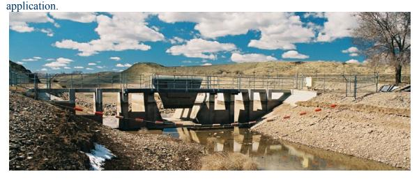
Amil gates have a trapezoidal gate-leaf and massive concrete buttresses. A large concrete saw was used to cut the buttresses from the floor of the structure. The Amil gate, the concrete buttresses, and one stop-log bay on each side of the of the buttresses were removed. A short concrete stem-wall was doweled into the floor of the check structure.
