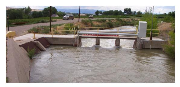
The base beam sets on a stepped stem-wall and the hoist channels are supported by vertical steel angle sections bolted to the inside of the outside concrete gussets. The assembled gate was placed into the modified structure using a crane.
