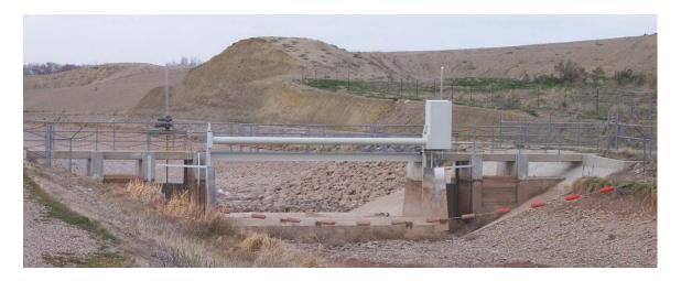
A 28-foot Langemann gate was installed in the open span. There is a small difference in water surface elevation across the gate-leaf, so that the hydrostatic pressures are nearly equal. Of the
