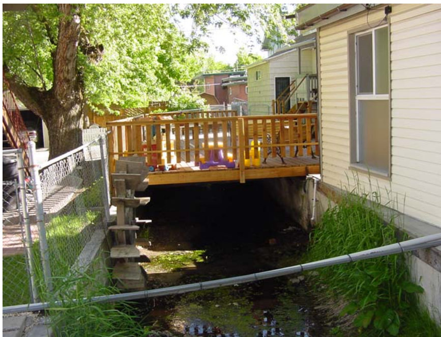
Fig. 12. Obstructions along a reach of the Logan Northfield Canal
