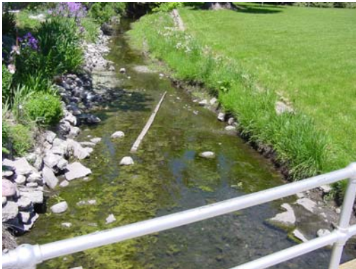
Fig. 4. Much weed growth and algae and narrow canal width (Logan Northwest Field canal)
