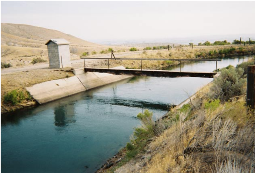
Photograph 6. At the South Canal site, flow depths varied from 3.5 feet to 5.5 feet during the 2003 irrigation season. Current meter measurements were made from the foot bridge.
