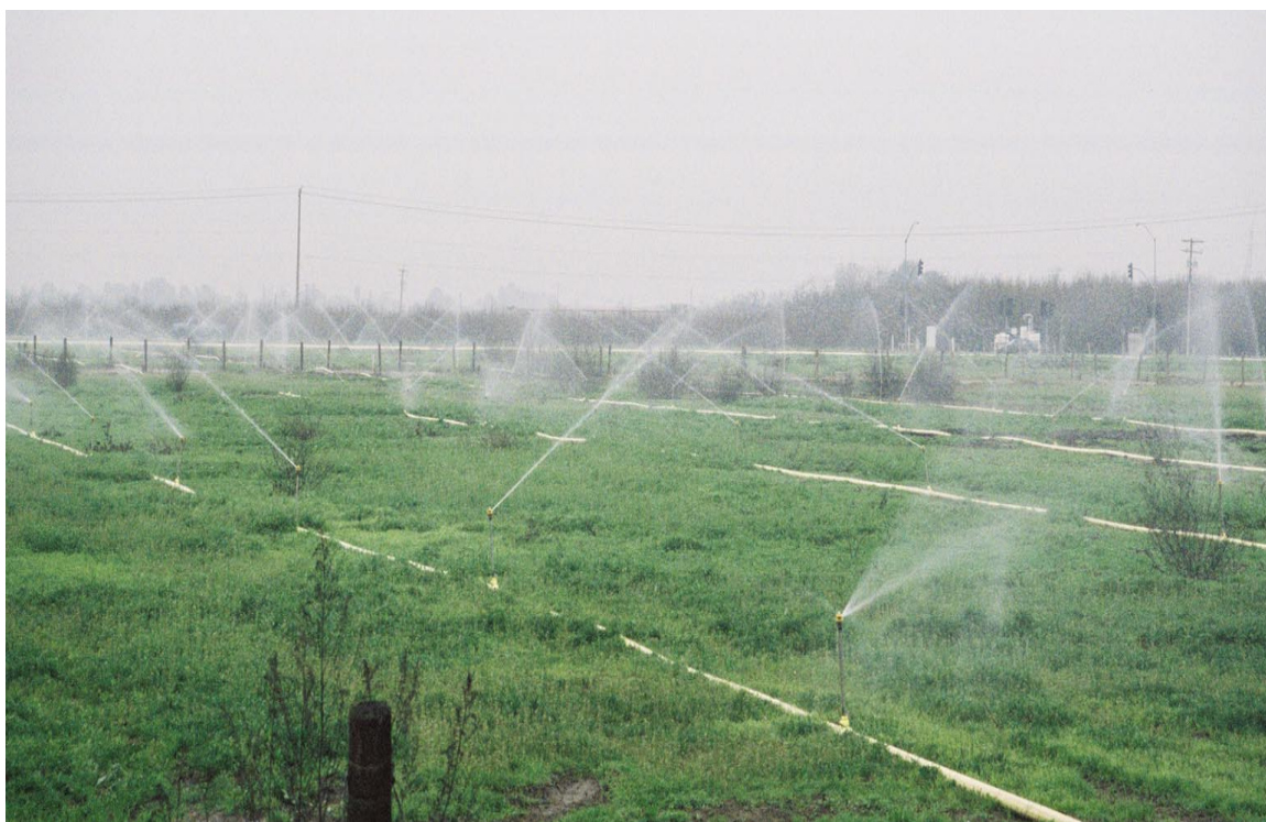
Figure 2 Certa-Set PVC irrigation piping portable solid set system in operation.
