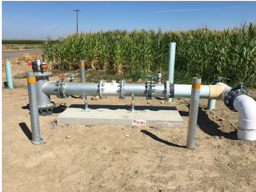
Wapato Irrigation Project – Farm turnout with butterfly valves
