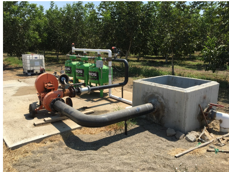
BCID (Tracy, CA) PTO pump, media tanks on pistachios
