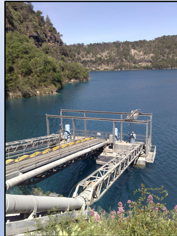
Blue Lake PS Mt Gambier, SA. Primary Lift Pumps
