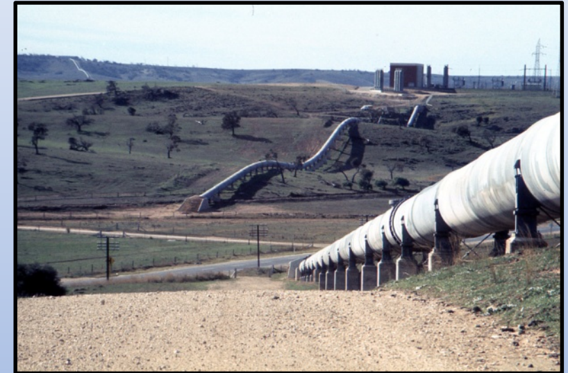
Murray Bridge – Onkaparinga Pipeline and No 3 PS (1973) 3 x 5,600 kW pumps (7,500 HP each)
