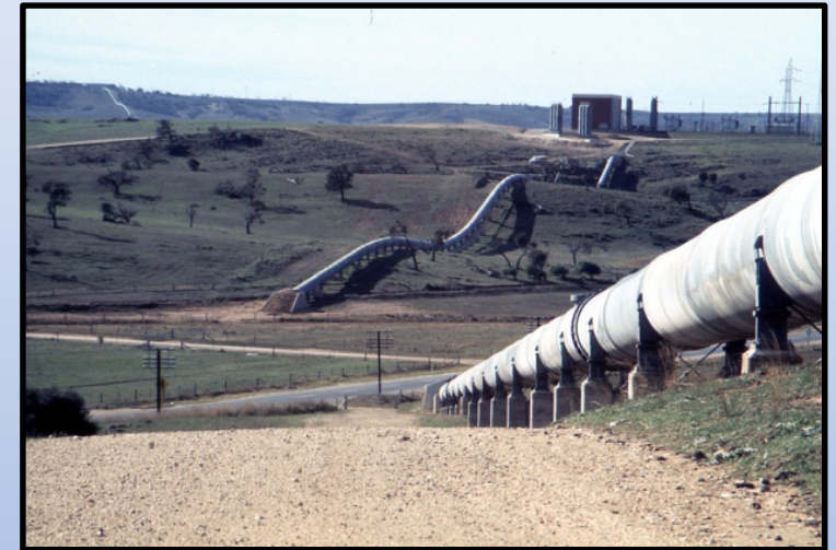
Murray Bridge – Onkaparinga Pipeline and No 3 PS 3 x 5,600 kW pumps (7,500 HP each)
