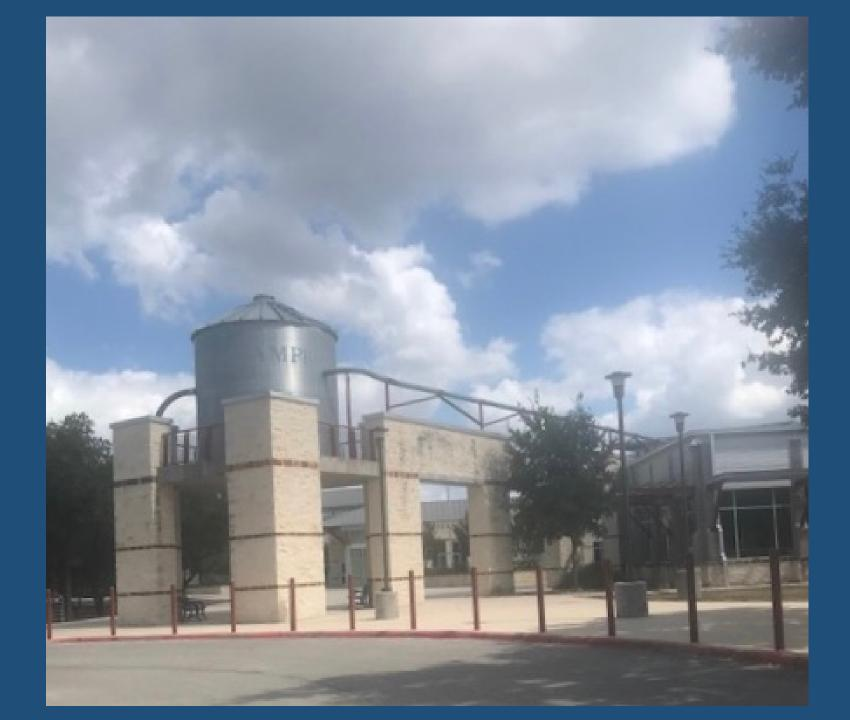
300,000 Sq. Ft Roof **5** Acres of Parking They collect from the roof, the HVAC condensate and the parking lot. Storage is a concrete pipe 8' x 8' x <sup>3</sup>/<sub>4</sub> of a mile long 1,800,000 gallons of Storage
