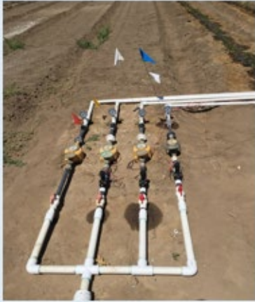
Fig. 2. Flowmeters with Valves (Tomato & Lettuce)
