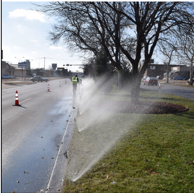
Before installation - Median 1
