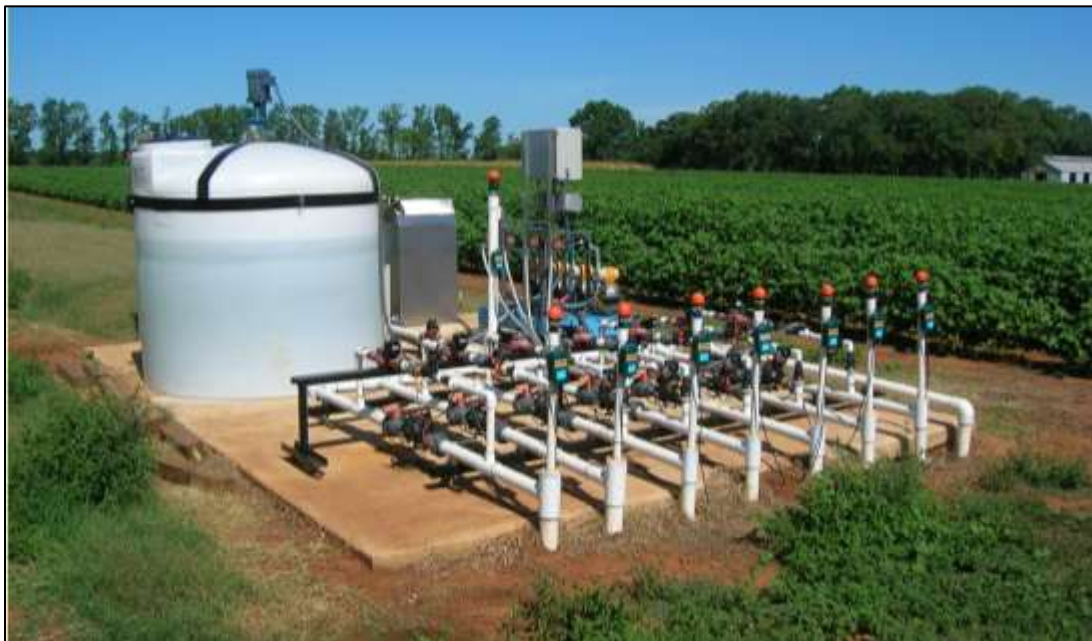
Fig. 2. Fertigation mixing tank, chemical injection pumps, and injection header for five replicated SDI fertilizer treatments and two irrigated buffer (guard) rows, Belle Mina, AL
