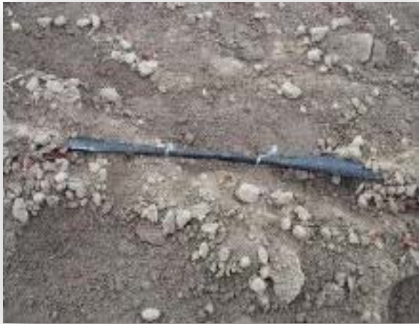
Figure 3: The term “jumpers” refers to the practice of inserting small diameter tubes in tape runs to reduce pressure buildup on extremely sloped terrain. Photo courtesy of Jim Klauzer, Clearwater Supply.
