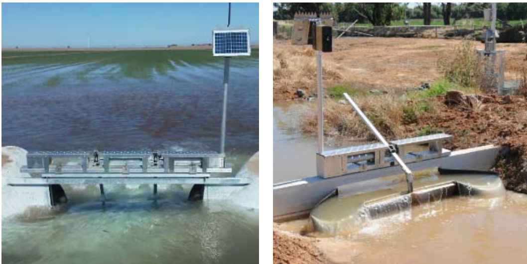
Figure 12 – Automated High Flow Surface Irrigation Systems
