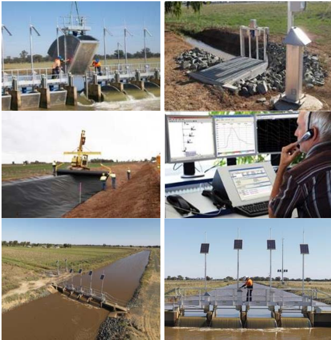
Figure 6 – Modernized Canals in Victoria's NVIRP Project
