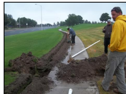
Irrigation modifications at Ford Frick Park
