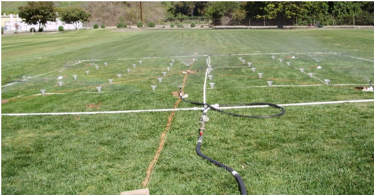
Figure 2. Test system with nozzles , catch cans, point of connection, water meter, and pressure gauge.
