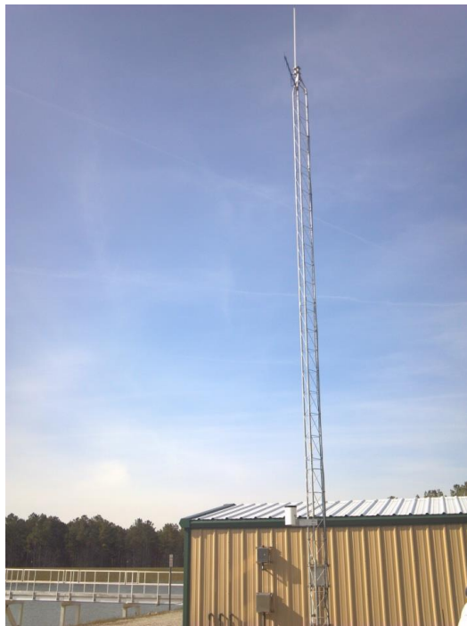
Figure 4. Communications Tower Installed at Remote Site
