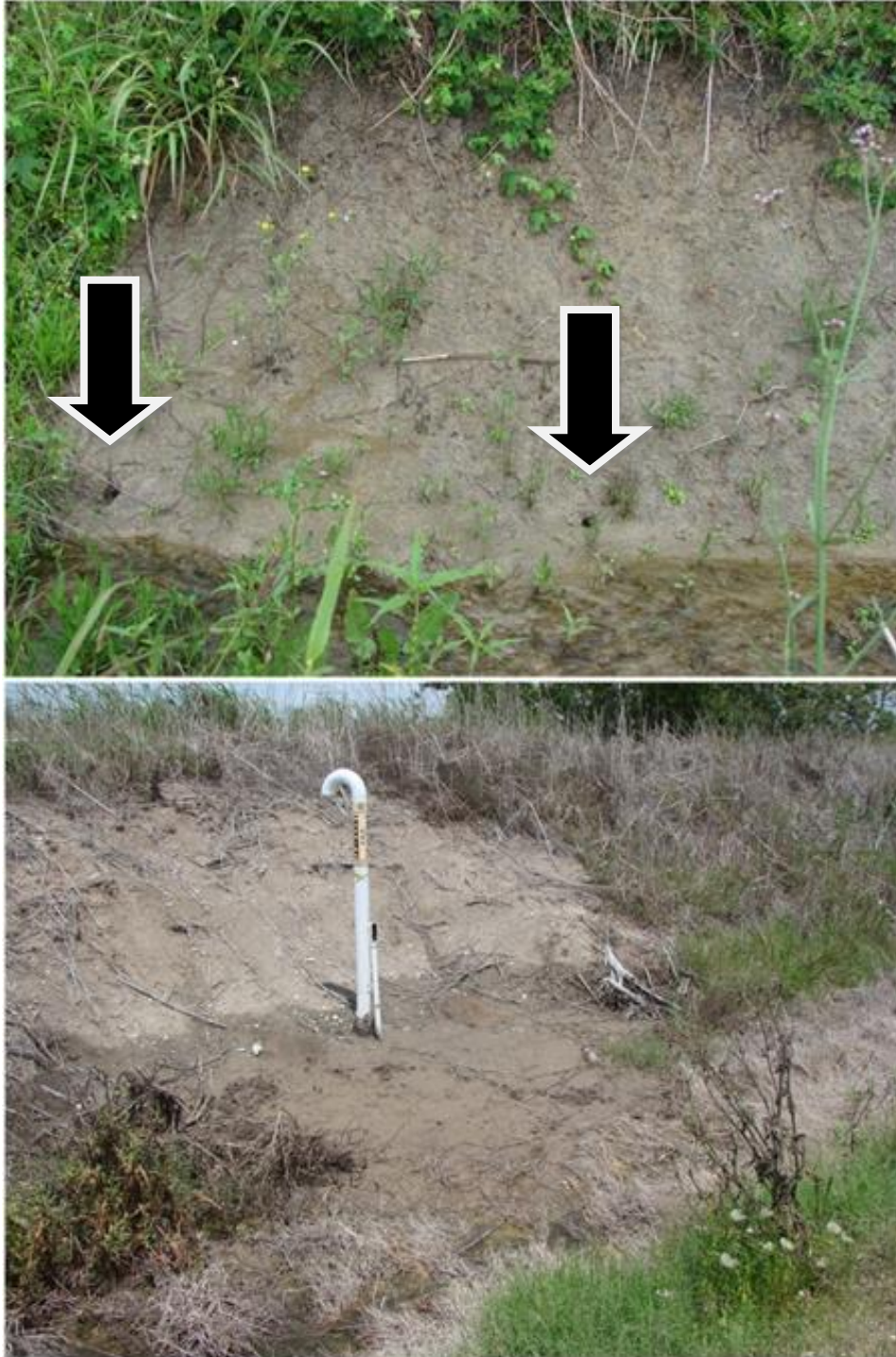
Figure 8. Seepage observed in canal embankment due to crayfish burrows (1S4, top), and pipe crossing (4S5, bottom) in the Texas case study. Arrows identify the point of seepage/leaks
