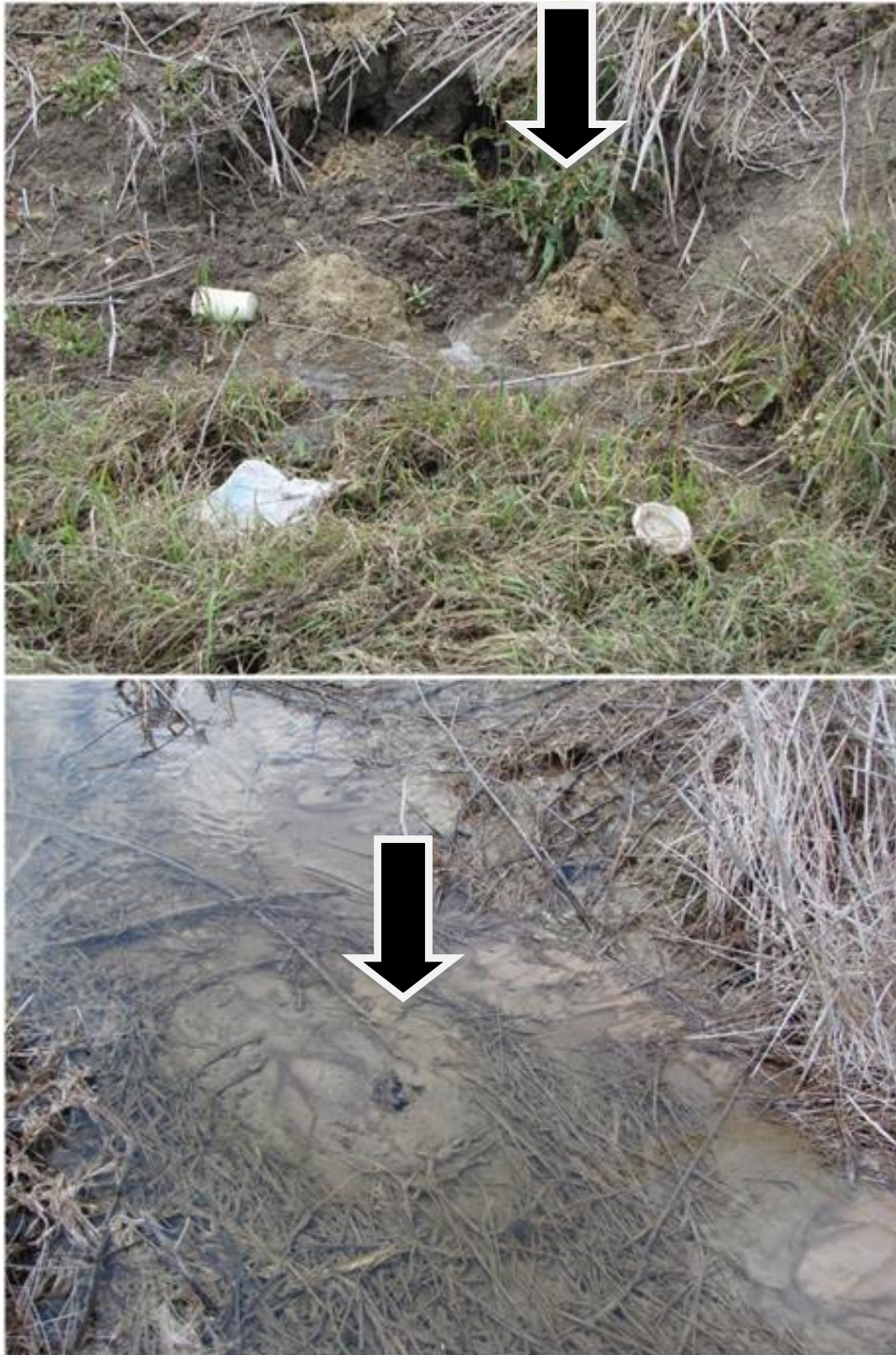
Figure 7. Seepage observed in canal embankment due to pocket gophers (4S7, top), and a crayfish burrow (4S5, bottom) in the Texas case study. Arrows identify the point of seepage
