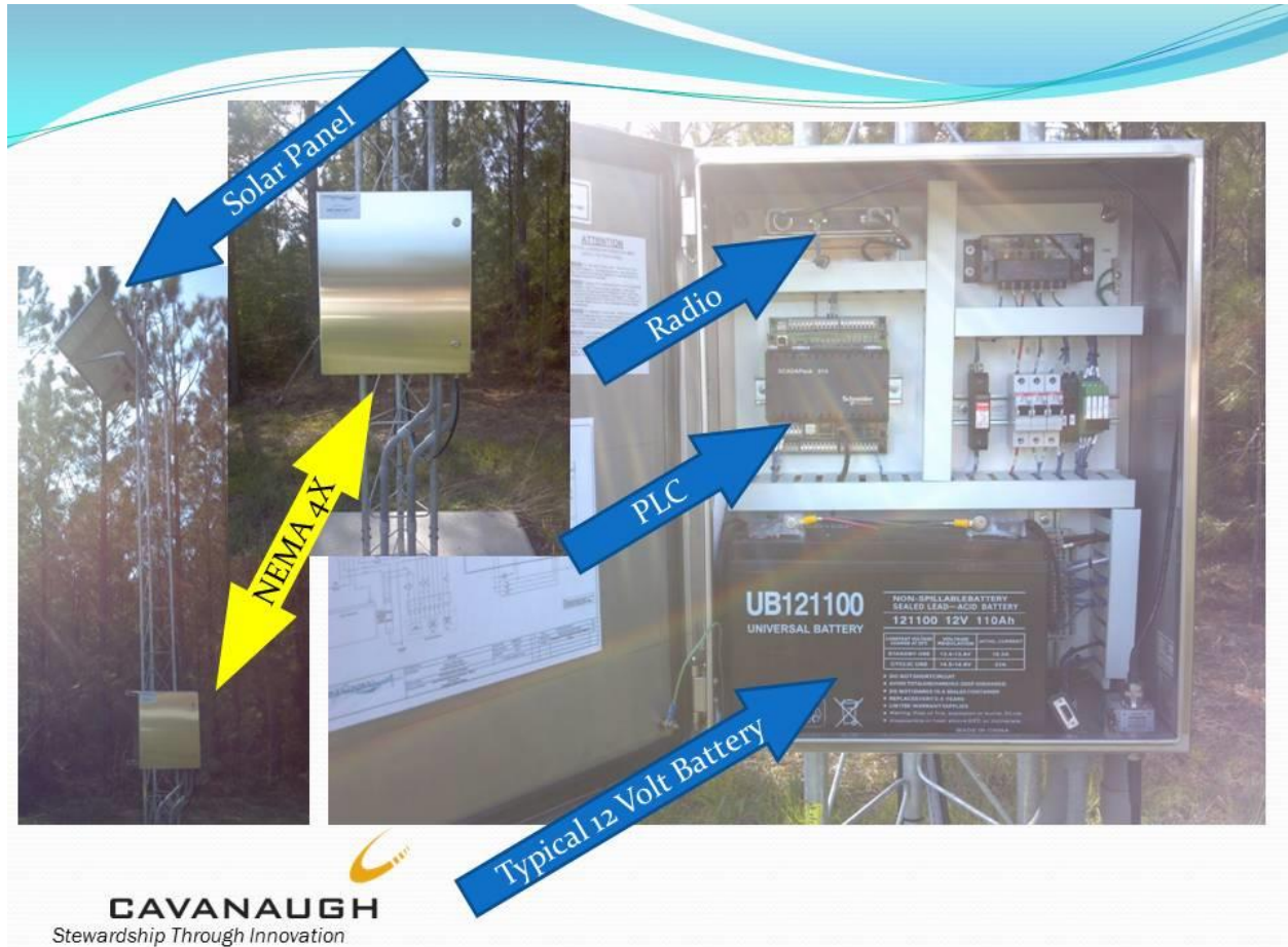
Figure 6. Typical Remote Irrigation Control System Installation
