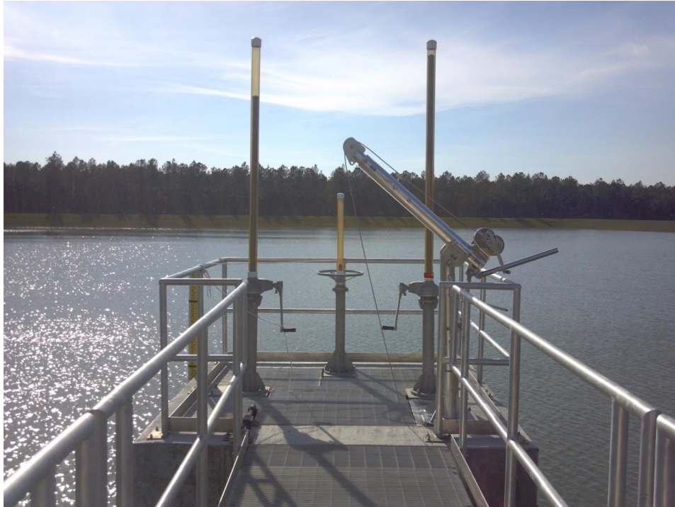
Figure 7. Inlet Control Structure at 32-acre Storage Pond Serving Surf City Irrigation System
