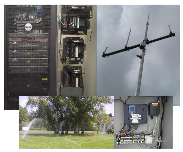
To truly be successful in implementing a Central Control System the buyer/operator must realize that a central control system is not merely an irrigation system that communicates but rather it is a communication system that irrigates. Why this distinction? Because communication technology is far more complex and difficult to implement successfully than irrigation control. Adding a radio to an irrigation controller does not provide the end user with an effective central control system.
