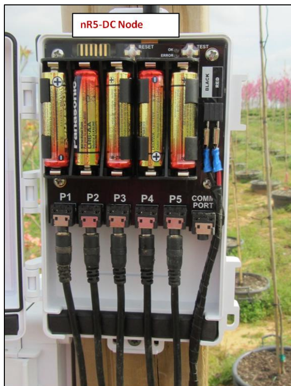
Fig. 3(b) The nR5 monitoring and control node, which provides local setpoint (sensor-based) control, in tandem with the 12V-DC latching solenoid (see Fig.4).
