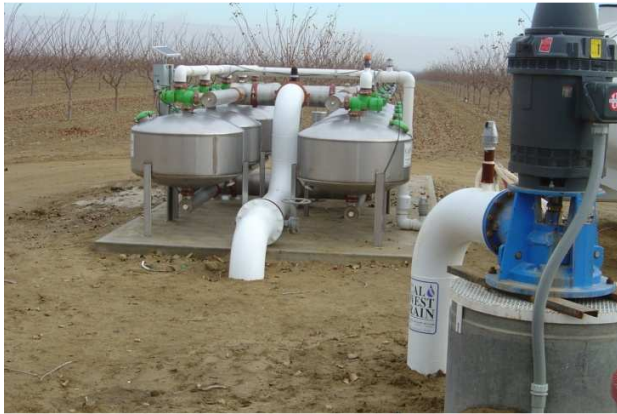
Figure 5: A well pumping water into sand media filters.
