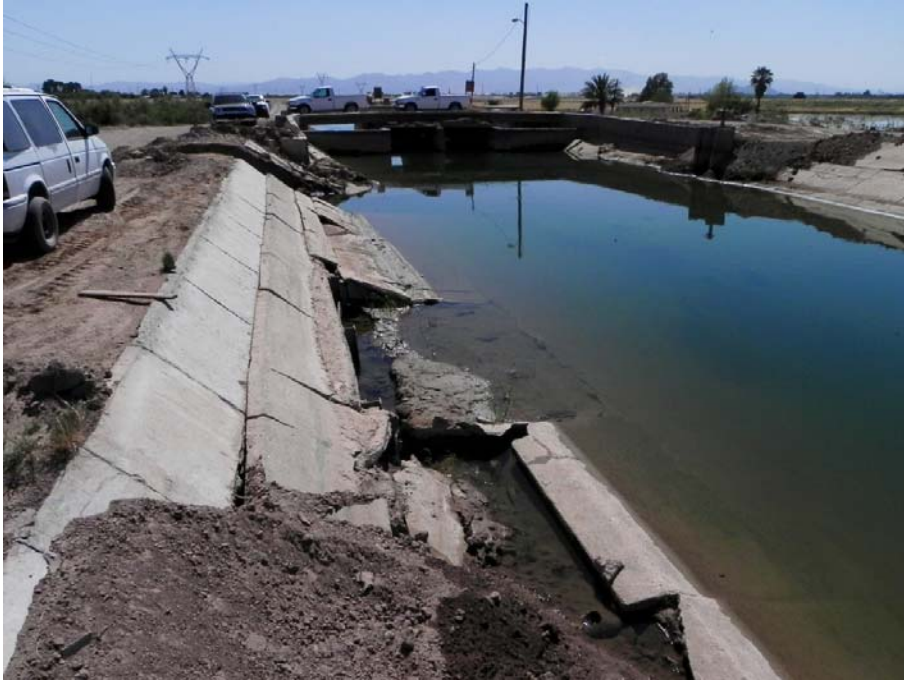
Figure 6. Damage to canal lining.
