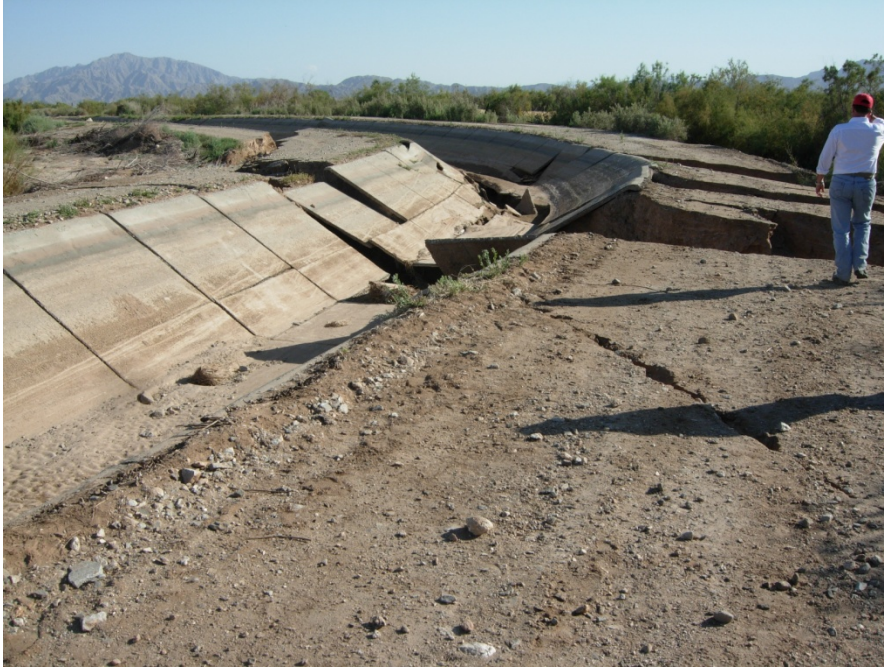
Figure 8. Damaged secondary canal.
