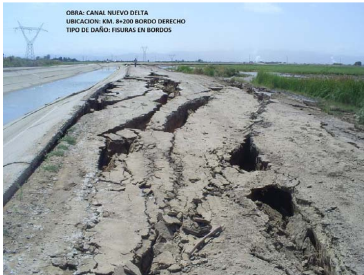
Figure 10. Fissures in the embankment road. Photo courtesy of CONAGUA.
