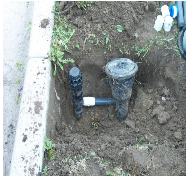
Figure 8 shows old impact sprinkler being replaced with new more efficient sprinkler.
