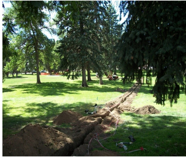
Figure 6: Installation of new irrigation system
