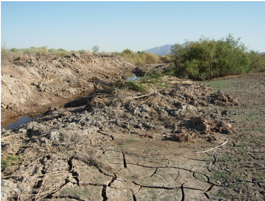
Figure 9. Drainage ditch that had collapsed and was partially excavated to provide limited remedial removal of salty water.
