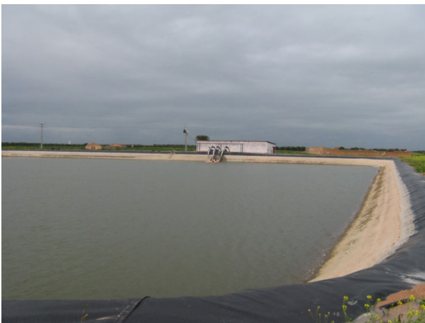
Figure 9. Water storage reservoir lined with a geomembrane. PIT, March 2009
