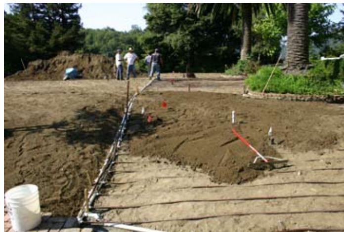
Figure 2. Adding soil over sub-surface system in Zone A
