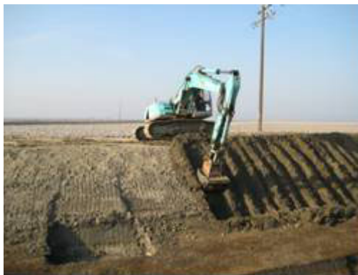
Figure 7. Compacting the canal banks on the James ID main canal with an MBW vibratory roller
