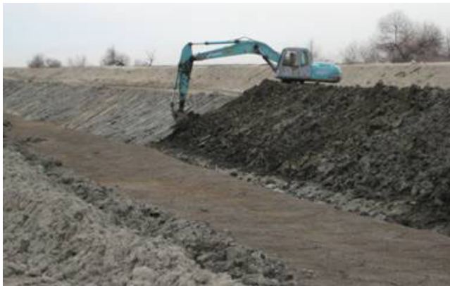
Figure 3. James ID Main Canal during side compaction
