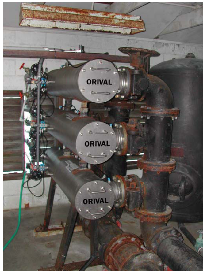
Figure 2. Three High Performance Stainless Steel Filters
