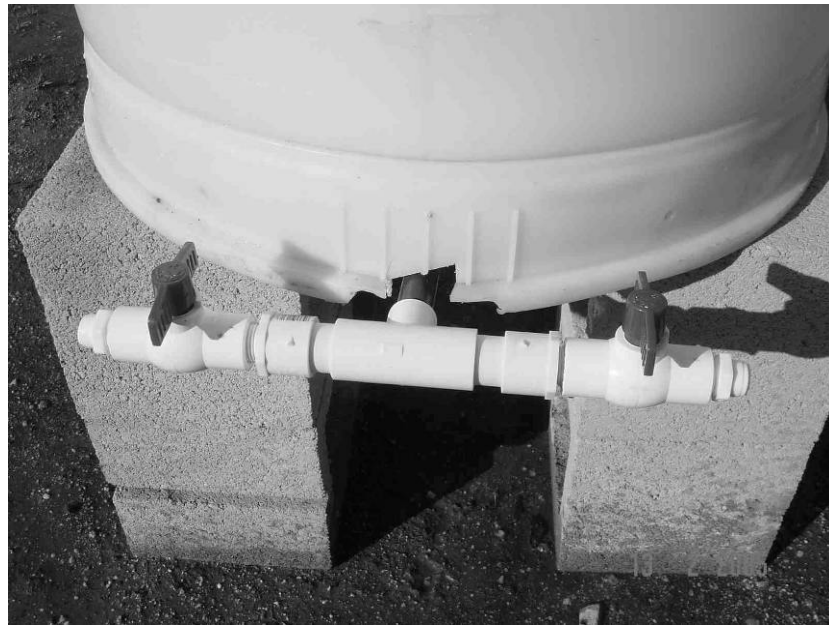
Figure 8: Base of the irrigation drum showing PVC outlet valves and connections.
