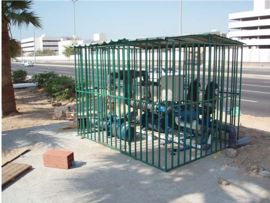
Figure11. The pump, filter, and control system housed in this enclosure are exemplary of the newest construction.
