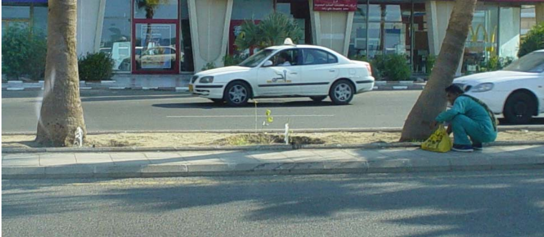
Figure 16. The “fountains” in the median are the result of the maintenance crew removing the bubblers from the risers during sprinkler operation. The bubblers are the black caps to the left of the fountains. It is assumed that the caps are then replaced at the end of the irrigation cycle, although several areas were observed with missing bubblers. This adapted approach to bubbler irrigation is the result of “cascading” operation and maintenance issues.
