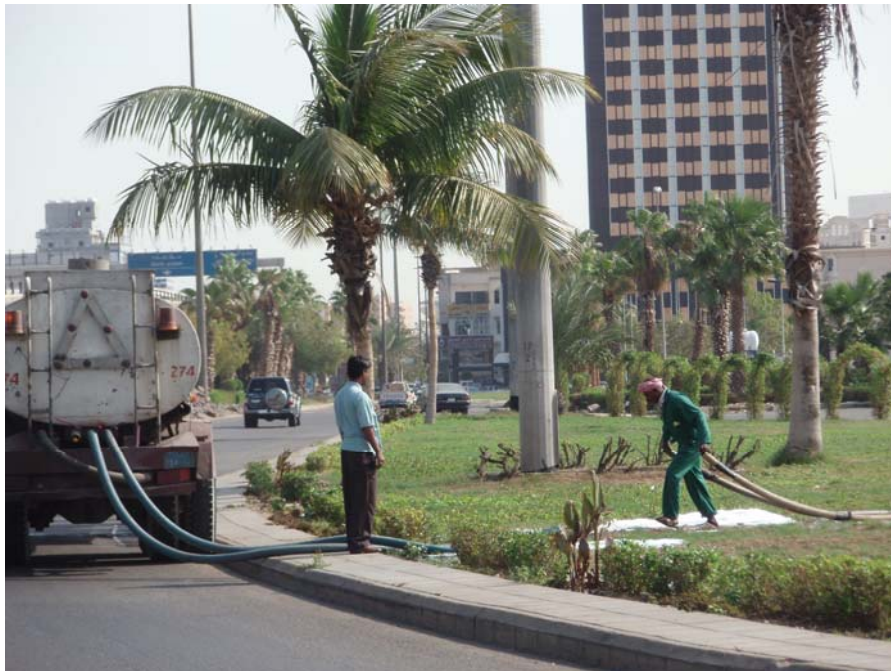
Figure 2. Some landscapes are surface or flood irrigated directly from tanker trucks as shown here.
