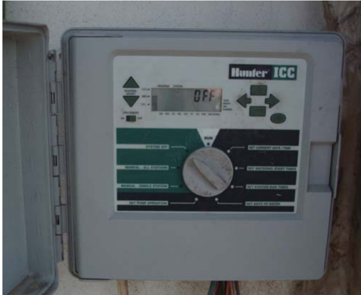
Figure 14. This irrigation controller is an independent controller not compatible with the central control system. Only a small portion of the 400 landscape irrigation sites are on the central system.
