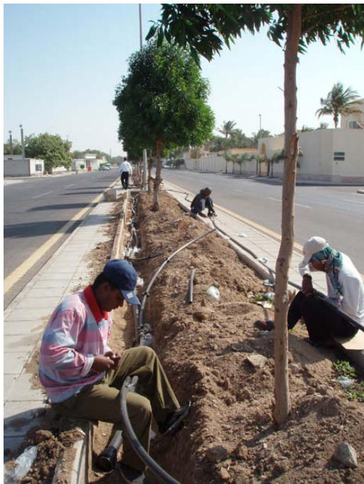
Figure 12. Workers shown here are installing bubblers that will be used to irrigation trees as well as understory groundcover.
