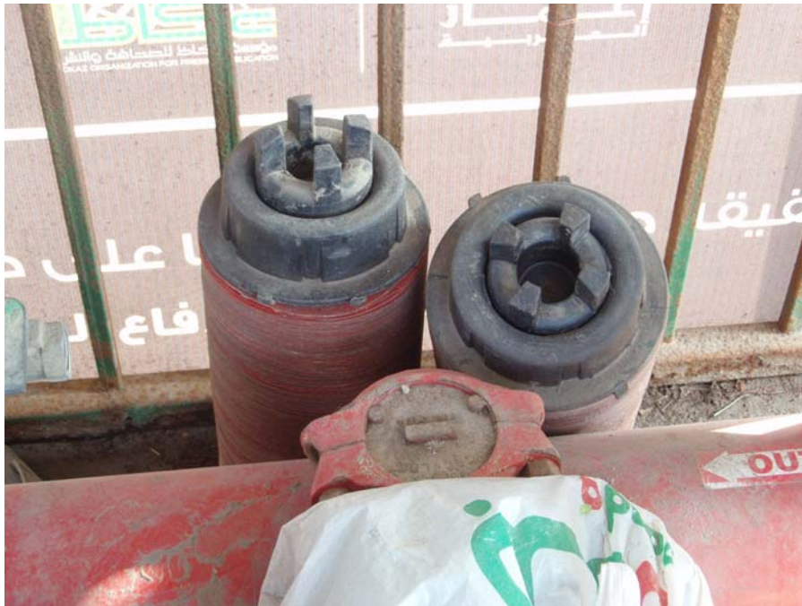
Figure 5. Filter elements are often removed by workers to increase flow and pressure downstream of the pump station. This, of course, aggravates plugging of emitters and orifices in other water emission equipment.
