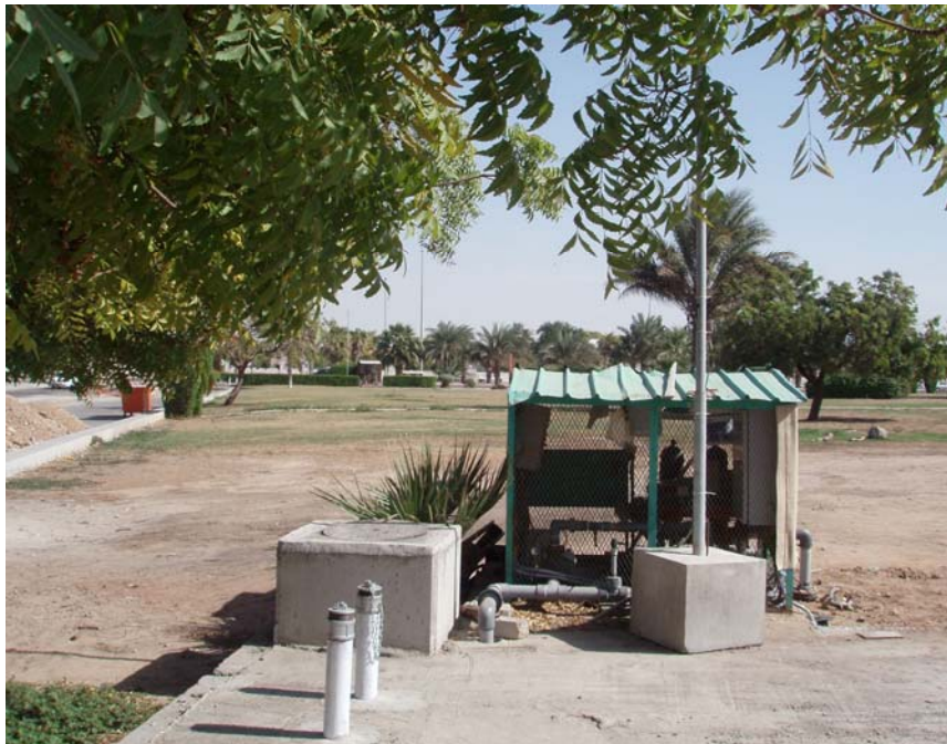
Figure 4. Pumps and filters are housed in expanded metal enclosures with a metal roof. The concrete tank holding 100 cubic meters of recycled water can be seen in the foreground. This site is centrally controlled and the antenna for the control system is set in the concrete block seen in the foreground.
