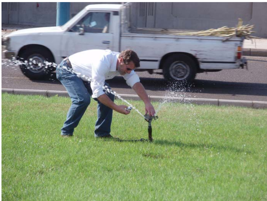
Figure 6. Pressures were measured to document dynamic pressures in the irrigation system. Low pressures were sometimes due to multiple laterals opened manually and simultaneously, thereby causing the pump to run out on the pump curve and produce inadequate pressures.
