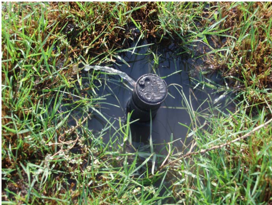
Figure 8. This operating sprinkler is clearly operating well below minimum acceptable pressures.
