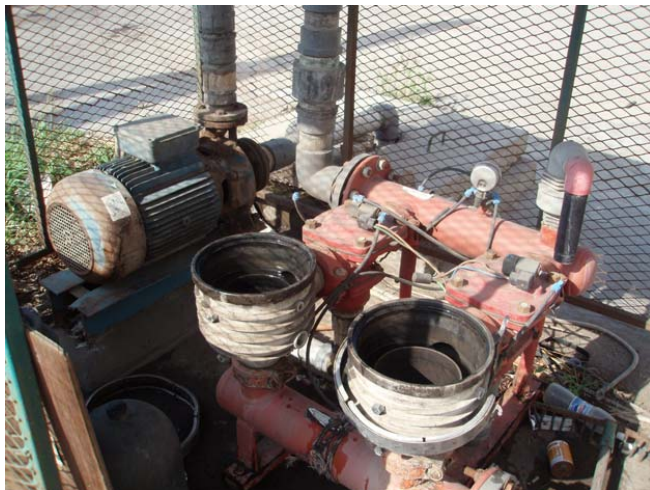
Figure 15. In the photo on the left above, the filters were disassembled to show that no filter elements were installed at the time of this site visit. In the photo on the right, the clogged filter element can be seen. This filter element was sitting off to the side -- uncleaned and unused.
