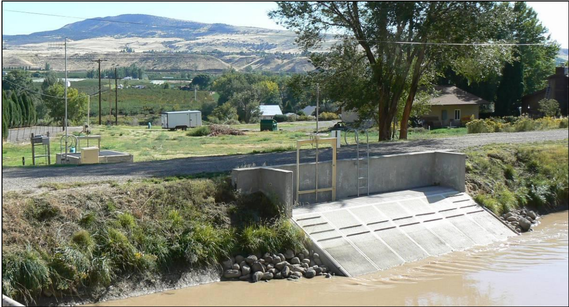
Figure 2: Palisade Pipeline Turnout from Highline Canal
