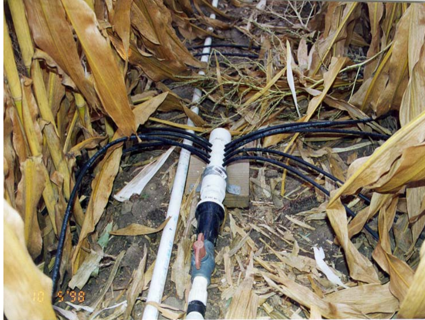
Figure 2. Flow divider with tubes used to deliver irrigation water to individual furrow basins.
