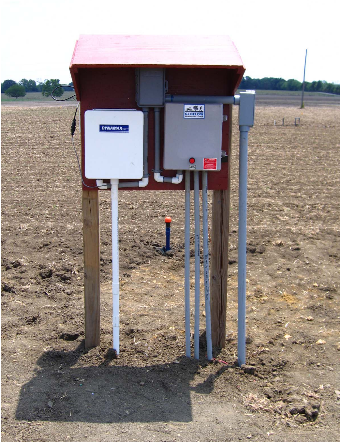
Figure 7. Finished field experimental system (Datalogger and Control box) at Black Belt Research and Extension Station, Marion Junction, Dallas County, Alabama.
