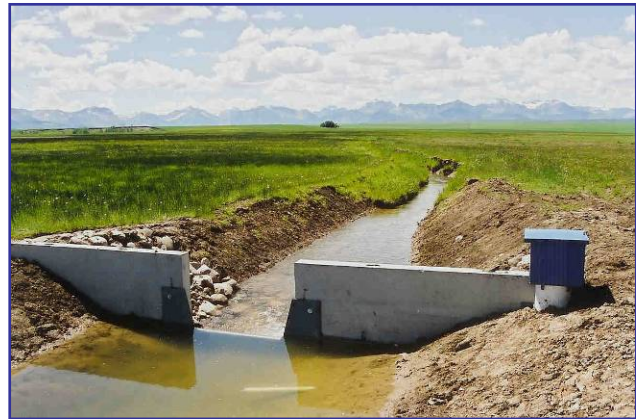
Figure 27: Return Flow Monitoring: Mountain View Irrigation District
