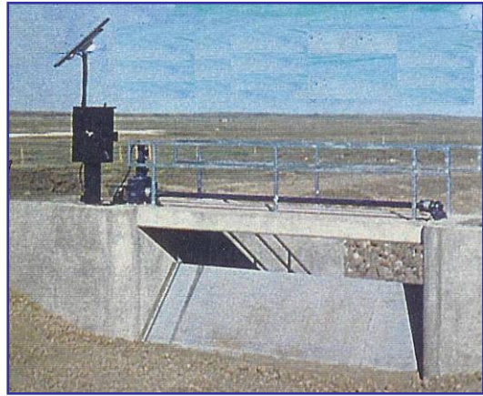
Figure 26: Automated (24VDC Solar) Check/Drop Structure
