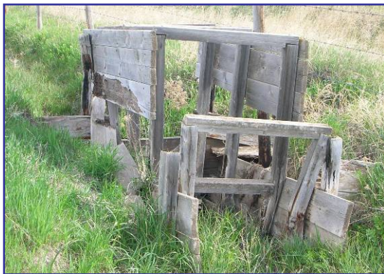
Figure 4: Old Wooden Control Structure
