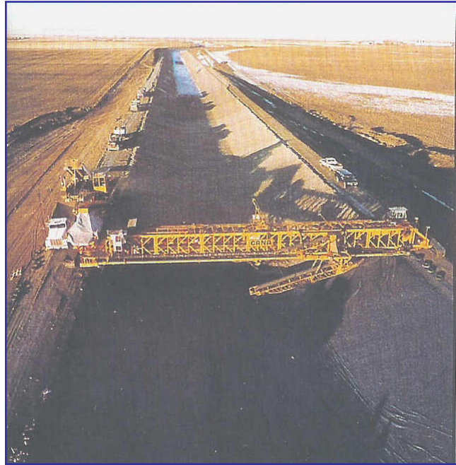
Figure 12: Canal Liner/Armour Placement Machine
