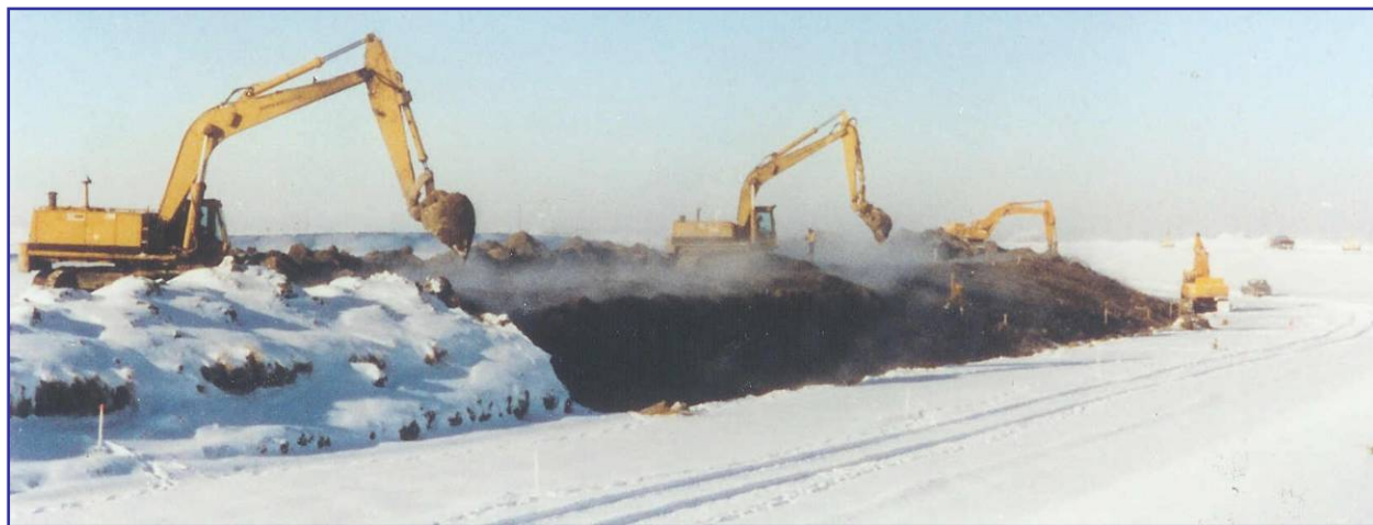
Figure 20: Winter Canal Construction
