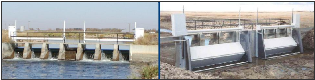
Figure 15: Langemann Gate in an 800 cfs (23 m 3 /s) Canal – Upstream & Downstream View
