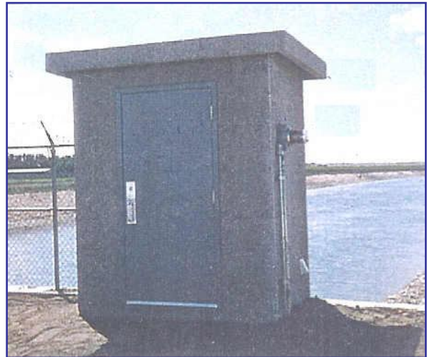
Figure 19: Precast Control Building
