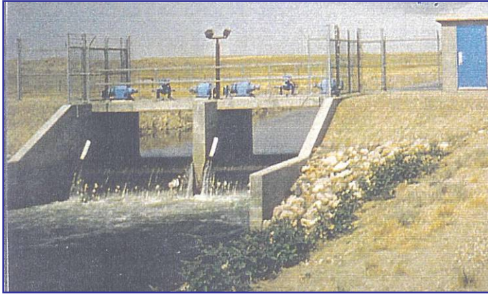
Figure 25: Automated (120VAC) Check/Drop Structure
