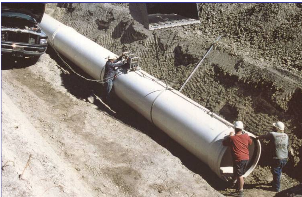
Figure 28: Installing Large Diameter PVC Pressure Pipe
