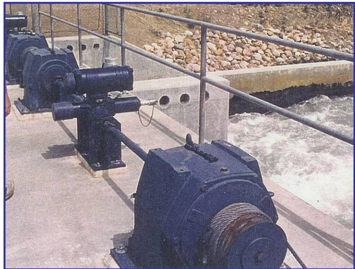
Figure 14: Large Drop Leaf Gate Hoist
