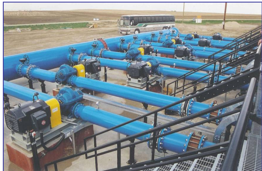
Figure 22: Centralized Irrigation District Pumping Station
