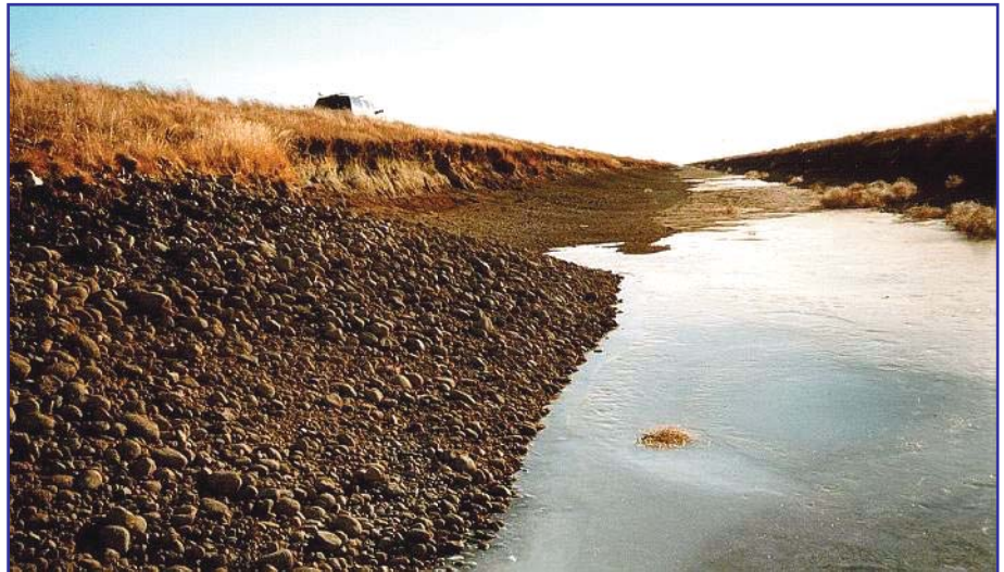
Figure 11: Armoured and Un-armoured Portions of a 20-Year Old Canal
