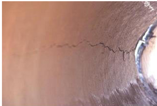
Figure 1. Water Hammer Damage in Concrete Pipeline
