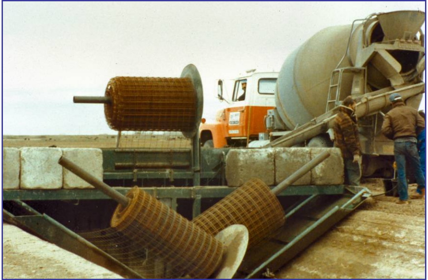
Figure 10: Installing Reinforced Concrete Lining
