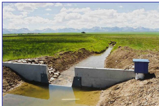
Figure 27: Return Flow Monitoring: Mountain View Irrigation District
