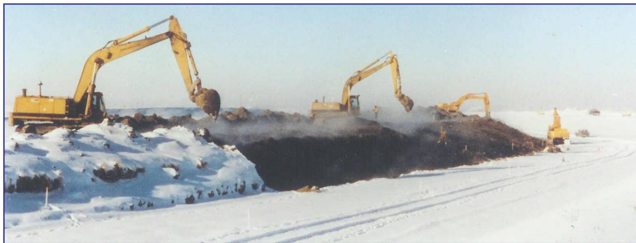
Figure 20: Winter Canal Construction
