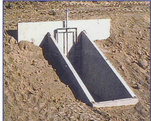
Figure 17: Precast Turnout Structure
