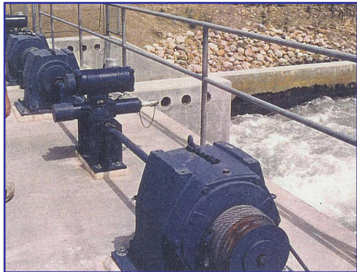
Figure 14: Large Drop Leaf Gate Hoist
