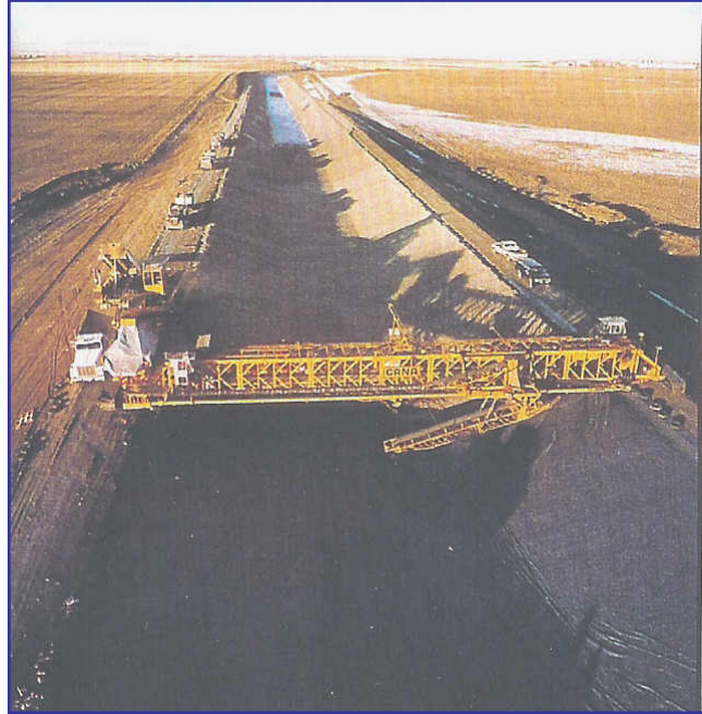
Figure 12: Canal Liner/Armour Placement Machine
