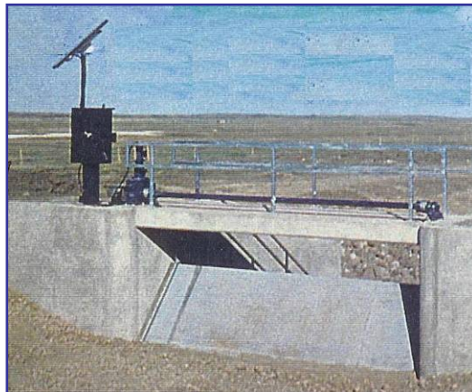
Figure 26: Automated (24VDC Solar) Check/Drop Structure
