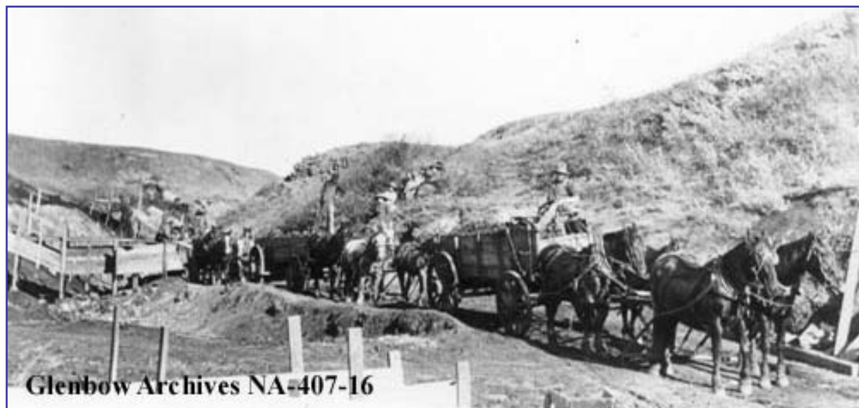
Figure 3: Irrigation Construction in the Early 1900's (Glenbow Museum Photo)
