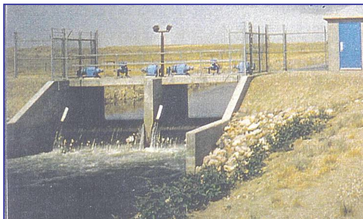
Figure 25: Automated (120VAC) Check/Drop Structure
