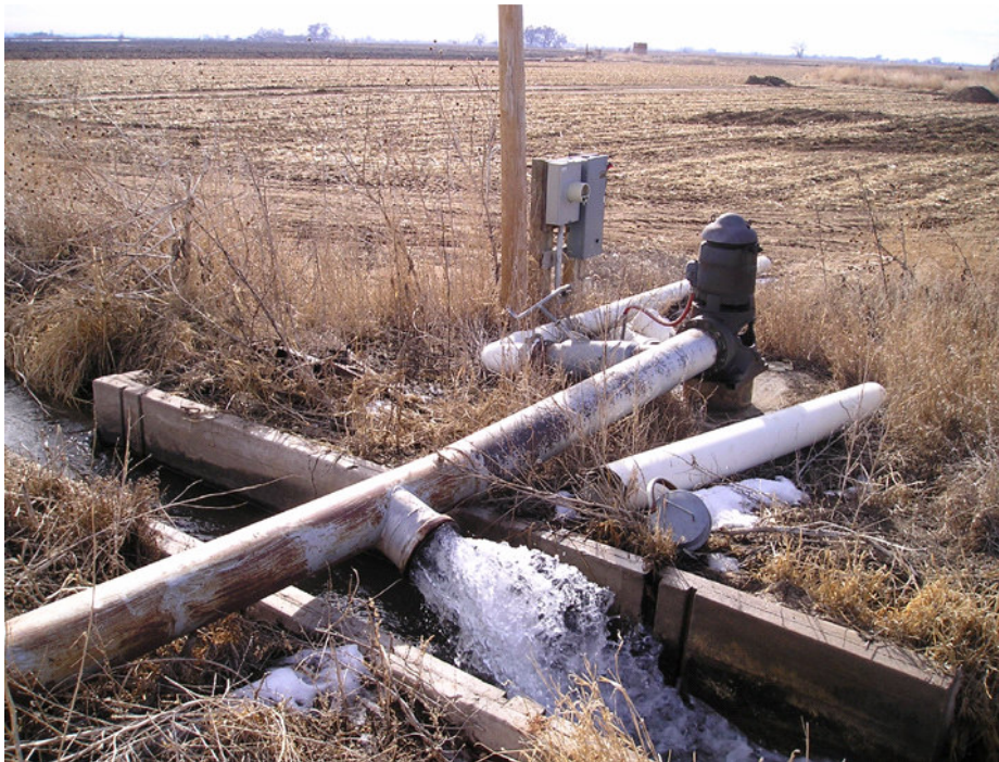
Fig. 3. Retiming well in operation. Water is pumped from the ground and is delivered to the river to cover stream depletions from irrigation well pumping. Sometime in the near future, stream depletions from the retiming well will occur in the river, and must be covered.
