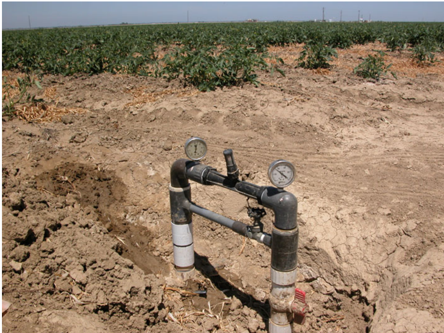
Figure2: Relatively larger injector servicing 24 drip lines.
