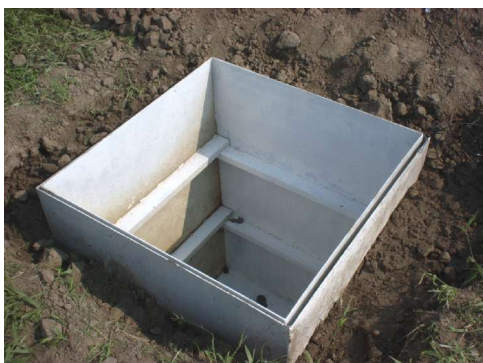
Figure 8. Install inner tank.
