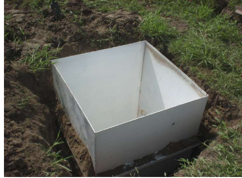
Figure 6. Backfill soil around outer tank.
