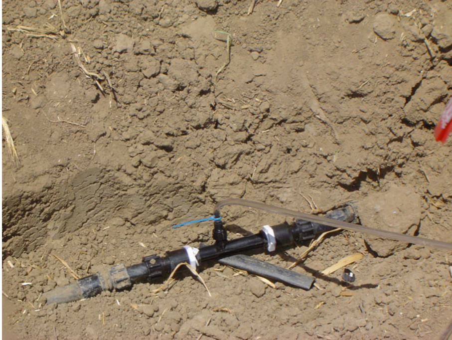
Figure 1: Single injector for each drip line.
