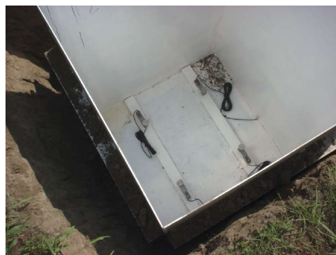
Figure 7. Install loadcells in outer tank.
