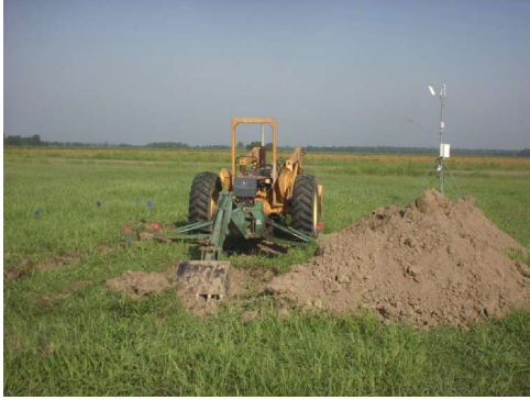
Figure 3. Choose location and begin excavation.
