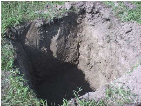
Figure 4. Remove soil and ensure bottom is level.
