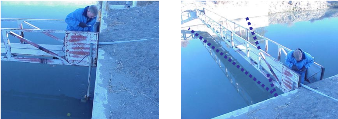
Figure 4. SonTek/YSI Argonaut SL installed in a canal
