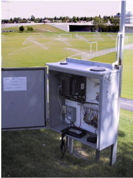
Figure 1: Central control system at Kingsland Dry Pond.
