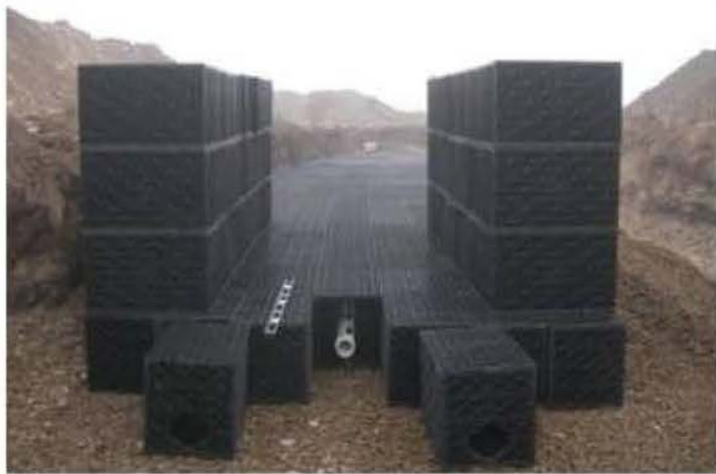
Raintanks being deployed
